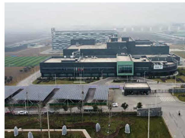
Our LEED Gold-certified Xi'an, China, Janssen facility with a 1 MW solar array installed in 2020.
