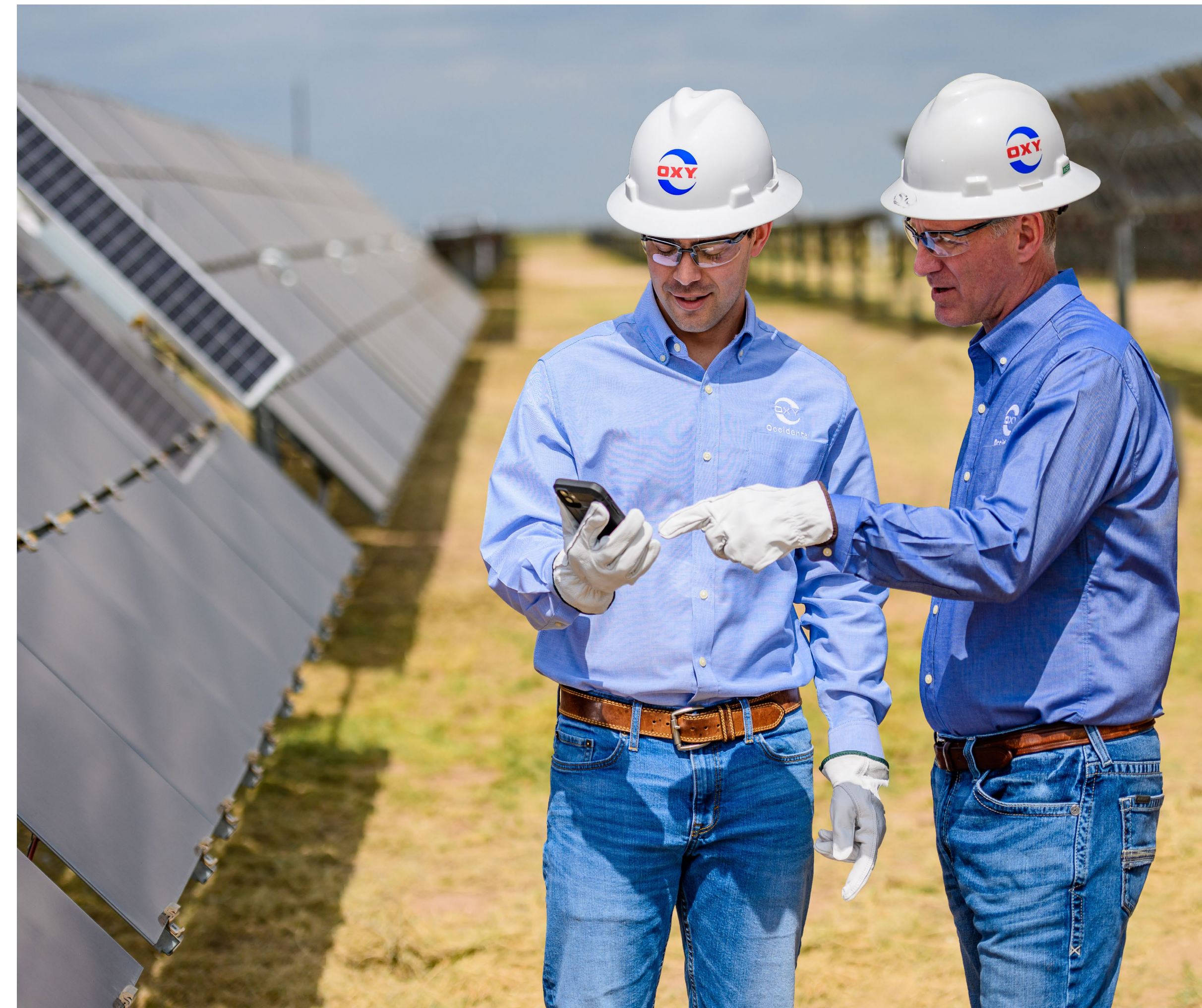
GOLDSMITH SOLAR PLANT, PERMIAN BASIN, TEXAS
