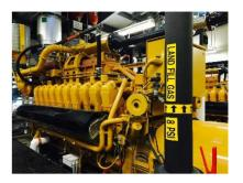
In 2014, GM took it a step further at Orion and Fort Wayne by investing in electrical generation equipment to convert landfill gas into electricity onsite, essentially allowing the company to act as its own utility. It saves on energy costs while reducing greenhouse gases. Gas that would have been flared at the landfill is now redirected into the facility to create electricity for building vehicles.
