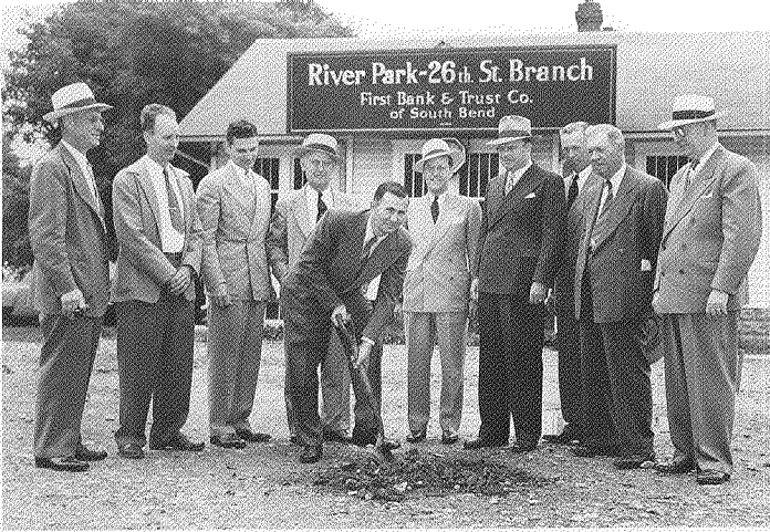
In 1947, ground was broken for a new office of the First Bank & Trust Company in South Bend's River Park neighborhood. The branch opened in 1948 at 2602 Mishawaka Avenue, and was the bank's second branch office and third location overall.
