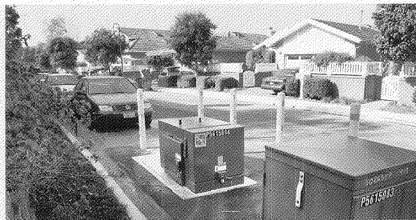
Storing Energy Locally: Batteries can be used locally in homes and neighborhoods to store energy from customers' distributed generators, such as in this neighborhood in Irvine where these transformers sit atop underground batteries.
