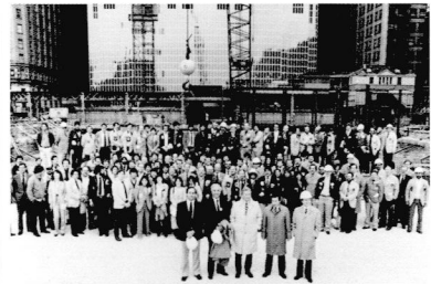
1981 CBOE breaks ground on a 350,000-square-foot building across the street from the Chicago Board of Trade.
