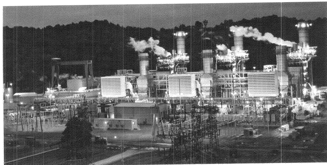
John Sevier Combined Cycle Plant Rogersville, Tennessee
