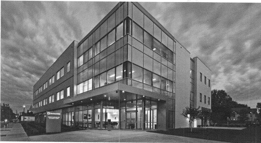
Cleveland Clinic Global Cardiovascular Innovation Center Cleveland, Ohio (LEED Gold Certified)
