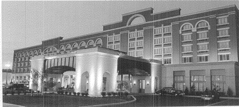
The Grande Hotel at Mountaineer
