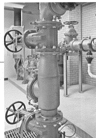
Ames Backflow Prevention Assembly Installation Fort Sill, OK
