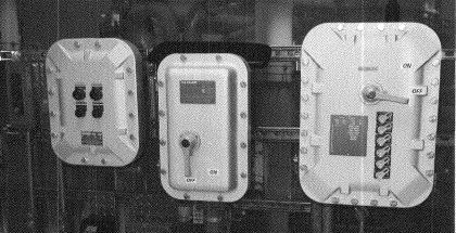
1 (Left to right) Killark DuraTech Controls, Nema Enclosures and Vergamate Breaker Protector Interlock Receptacle
