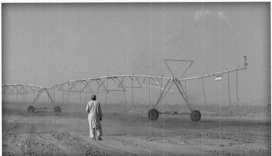
Zimmatic center pivot installation project near Kandahar City, Afghanistan.
