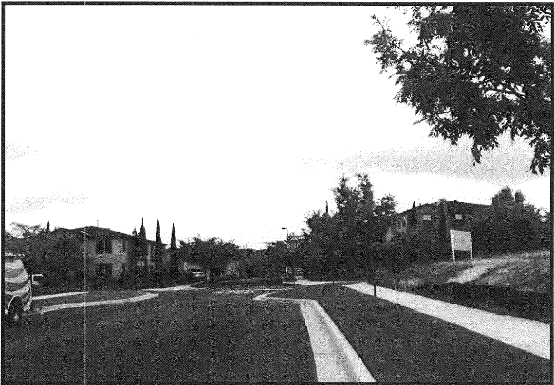
Looking North along Cottage Drive
