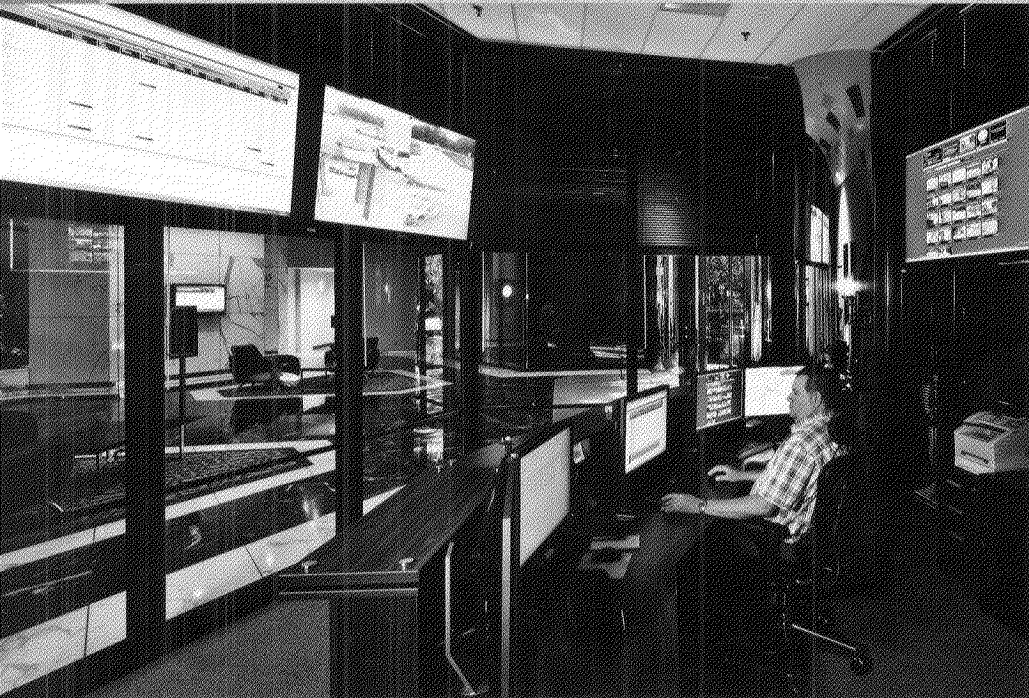
EXCO's Field Operations Control Center
