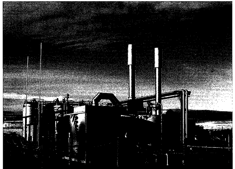
At Western Water's wastewater treatment plant in Melton, Victoria, a C200 microturbine burns biogas from the anaerobic digester to produce 1,700MWh of electricity each year. The electricity offsets the plant's overall power consumption by an estimated 60 percent.
