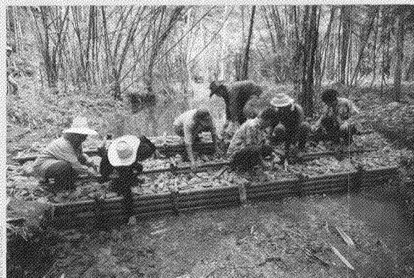
Villagers in Ratchaburi, Thailand, build a check dam
