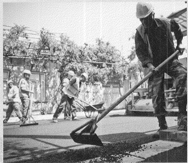
ADB has supported infrastructure upgrades in Adigeni
