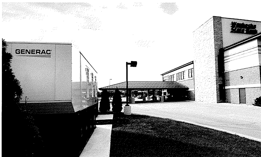
Commercial generator backing up a bank.
