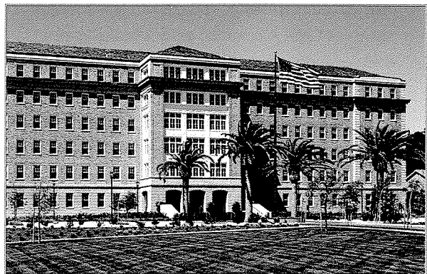
Lease-up is continuing at Presidio Landmark, the adaptive re-use of a former military hospital into 161 upscale apartments located within the Presidio National Park in San Francisco.
