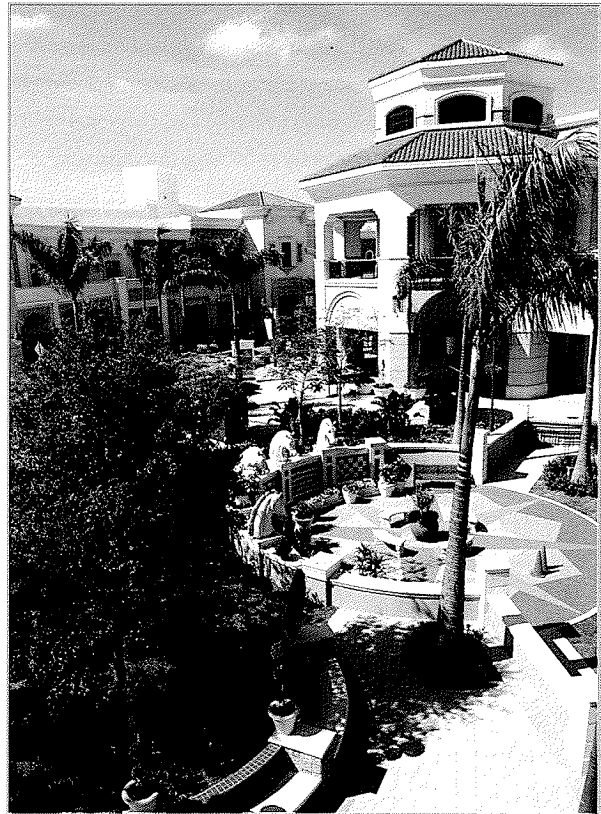
The 511,000-square-foot Village at Gulfstream Park is an open-air lifestyle center in Hallandale Beach, Florida, featuring dining and retail, and anchored by Gulfstream Park racetrack.
