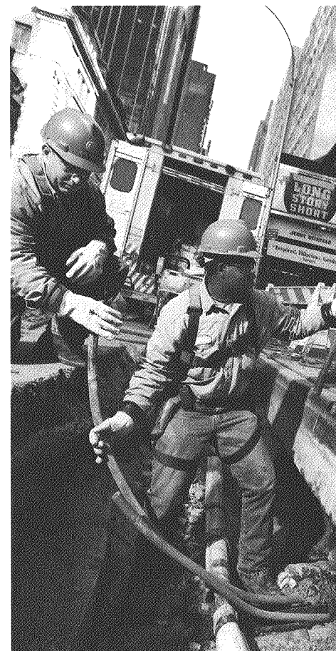
John Adorno, distribution splicer, and Russel Williams, distribution mechanic, upgrading service.
