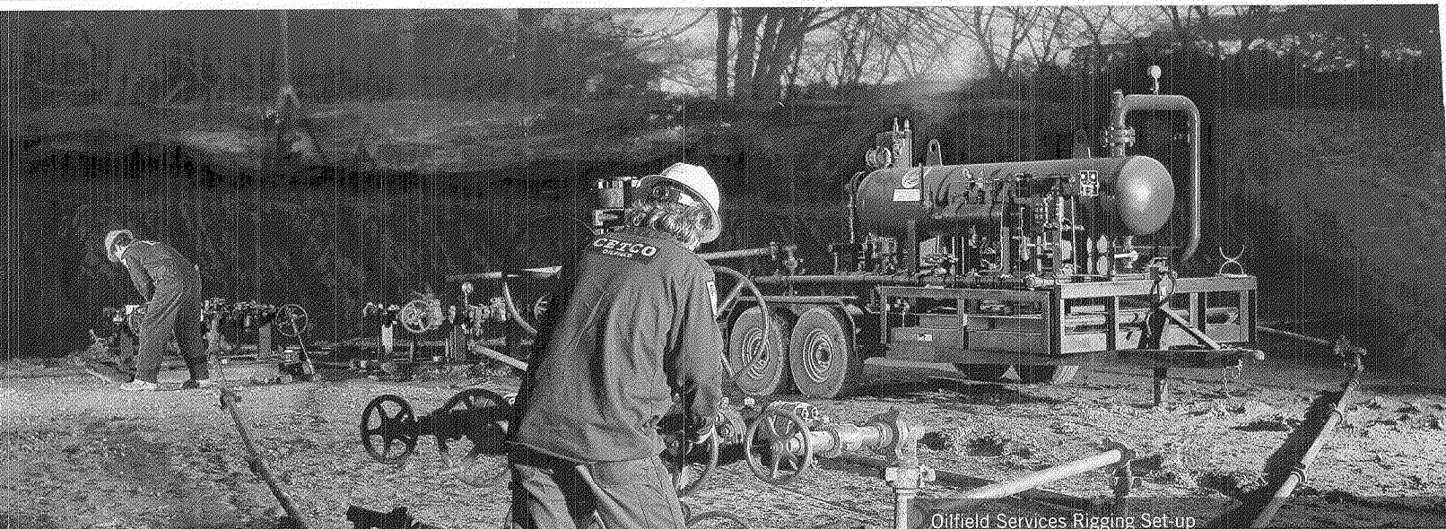
Oilfield Services Rigging Set-up
