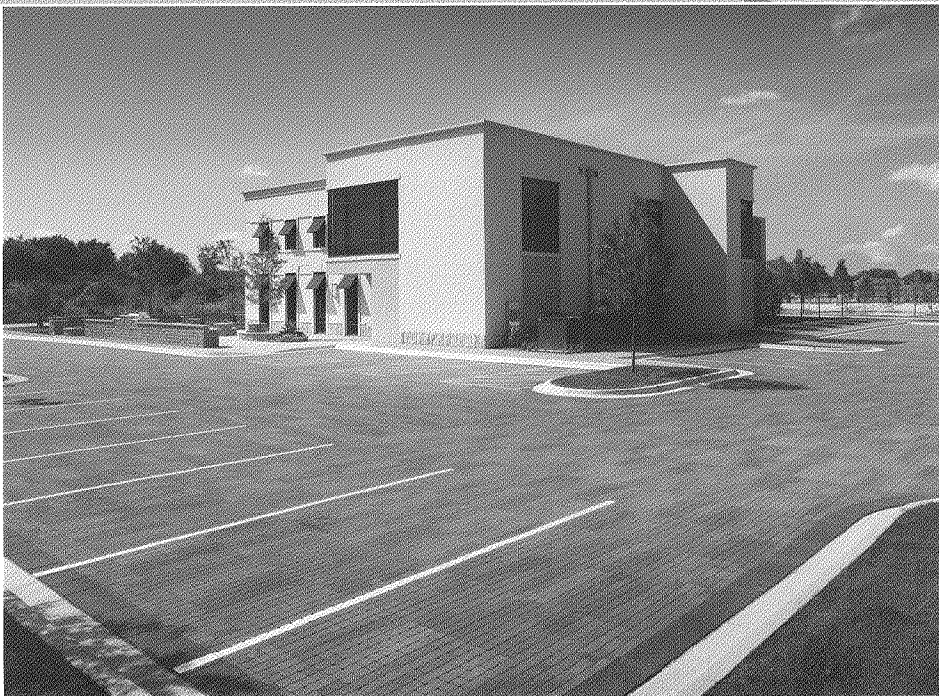
Below: Oldcastle Building Solutions provided a variety of products in the construction of a new Northfield Block office, north of Chicago, Illinois. CRH's Trenwyth masonry products provided both exterior and interior finishes while Oldcastle hardscapes were used for both the interior flooring and exterior permeable parking applications. Allied Building Products supplied drywall and roofing materials and other components to complete the project.
