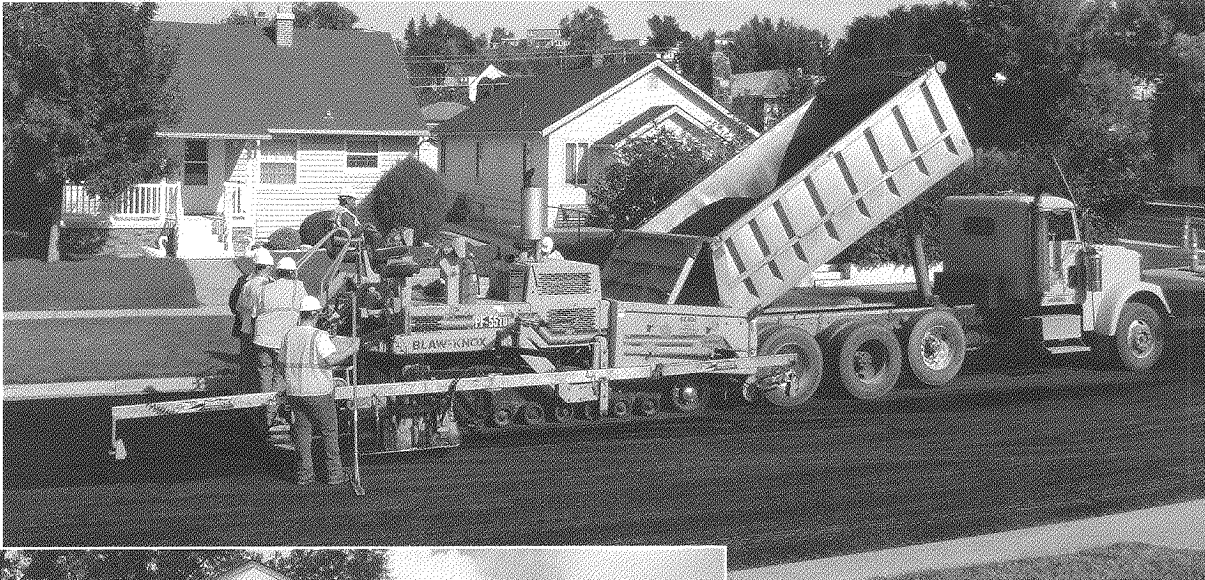
Above: In the US, Oldcastle Materials has pioneered the use of warm mix asphalt (WMA) which requires 15-30% less energy than traditional asphalt. Shown here is the first use of WMA in the state of South Dakota, laid by CRH subsidiary Hills Materials, at a residential neighbourhood in Rapid City. With over 100 WMA plants, CRH/Oldcastle produces circa 5 million tonnes per year.
