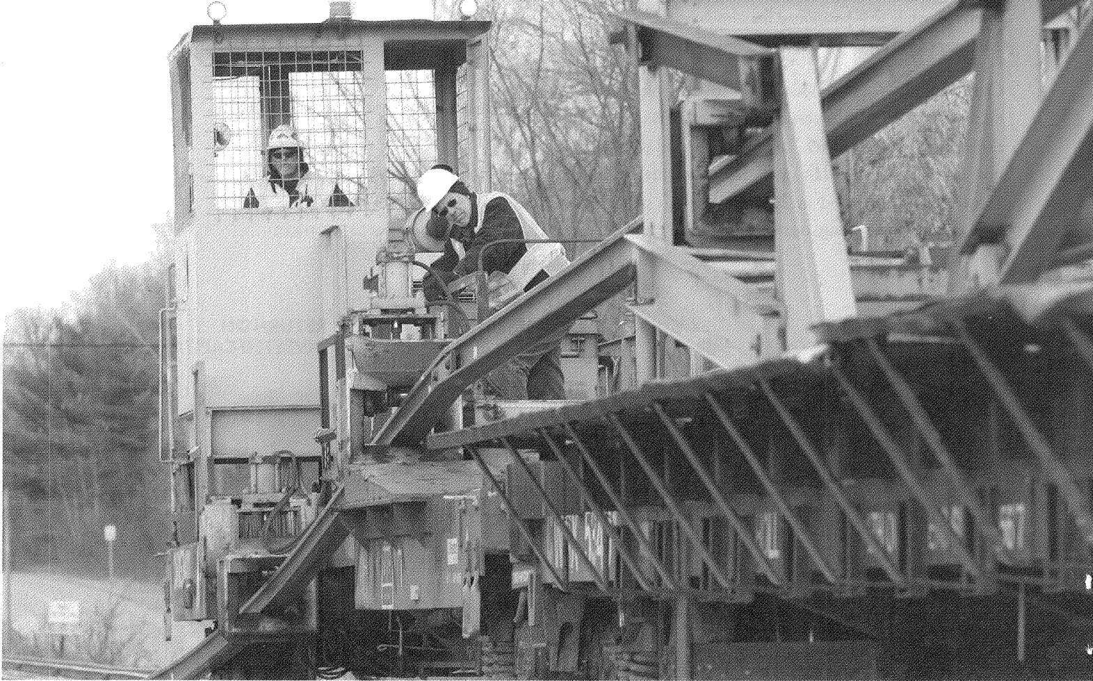
L.B. FOSTER WORK TRAIN UNLOADING CONTINUOUS WELDED RAIL AT JOBSITE ▼
