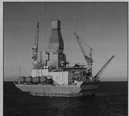
Orlan Platform, offshore Sakhalin Island, Russia
