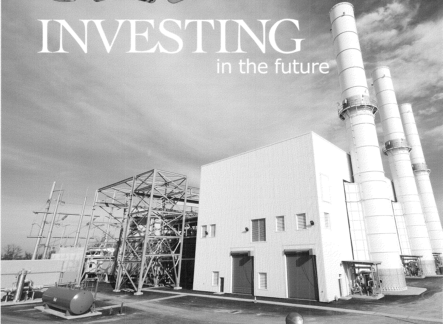
York Energy Center
