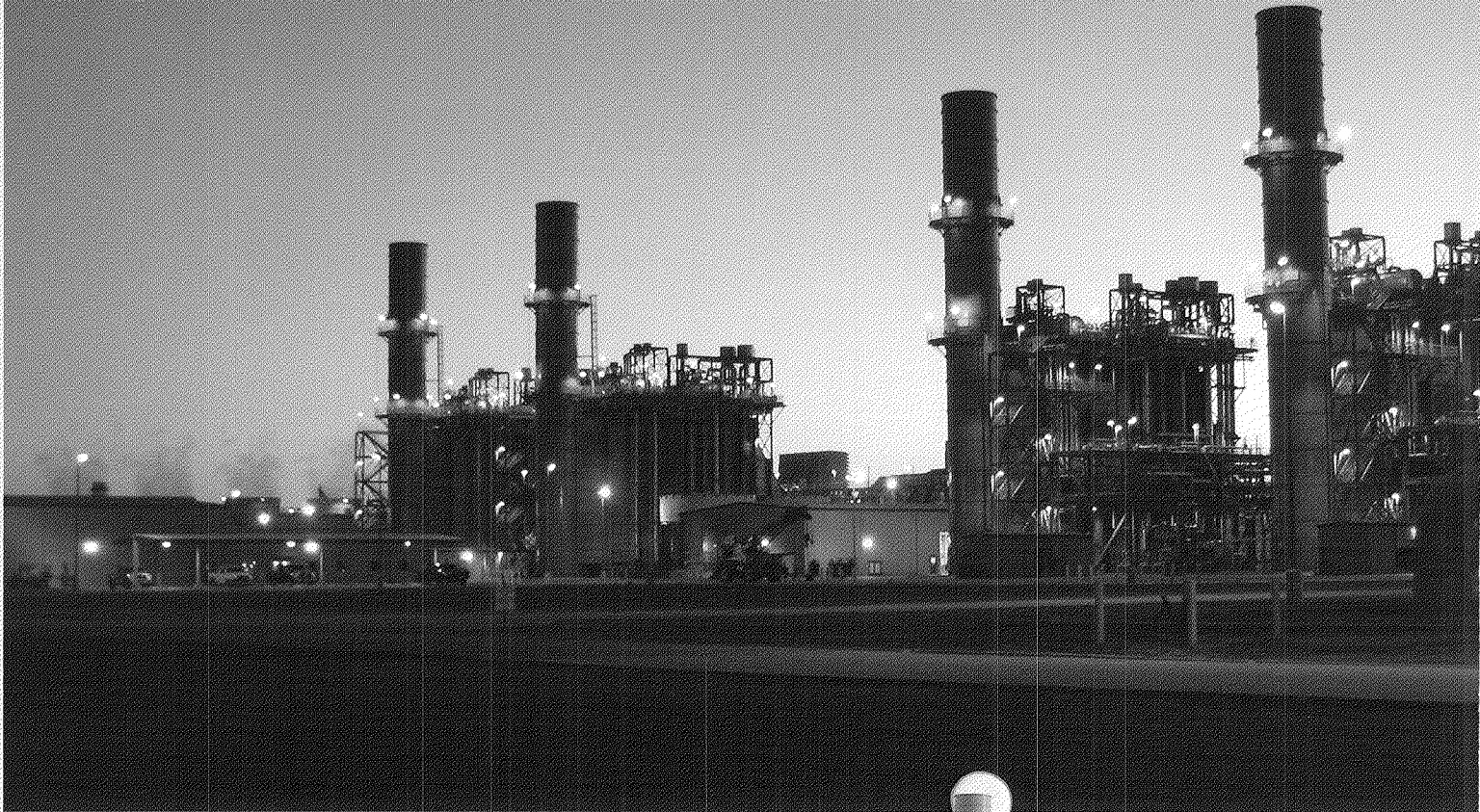
Freestone Energy Center
