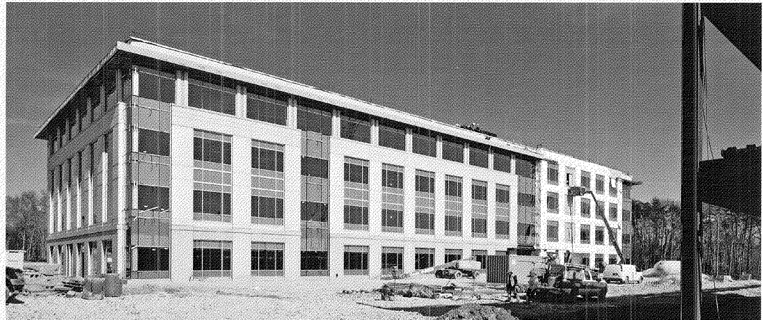
430 NATIONAL BUSINESS PARKWAY • UNDER CONSTRUCTION NEAR FORT MEADE
