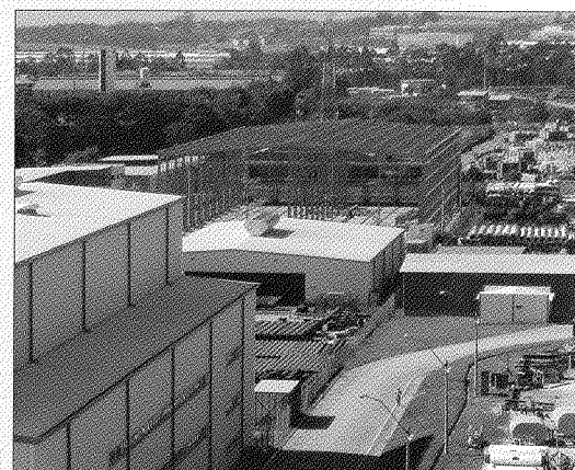
Construction of second Finish Machine Building
