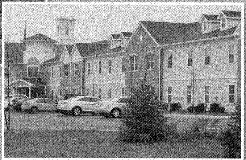
Chambersburg Senior Housing Project
