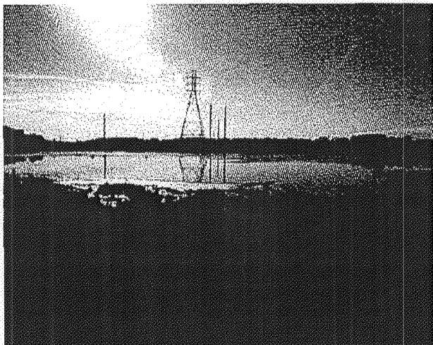
A surface impoundment in Georgia.
