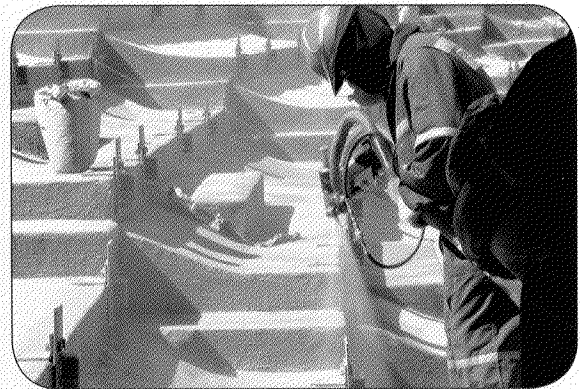
Polyurea application inside stadium
