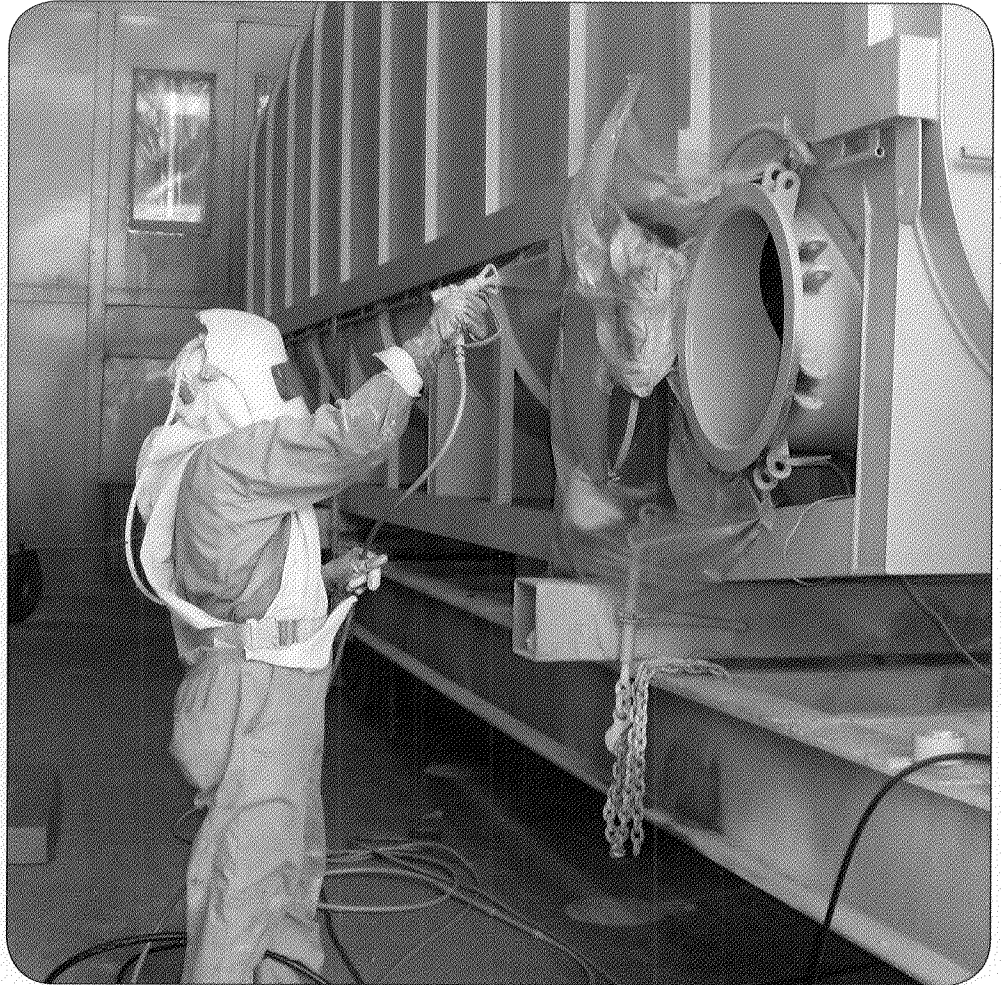
Atlas employee applies chemical coating inside tank
