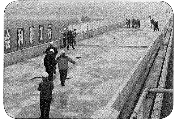
Beijing-Shanghai High-Speed Railway project
