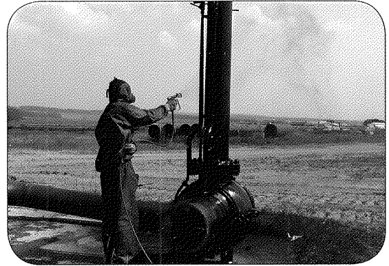
Spraying protective coatings on oil pipelines both above and below ground in Russia
