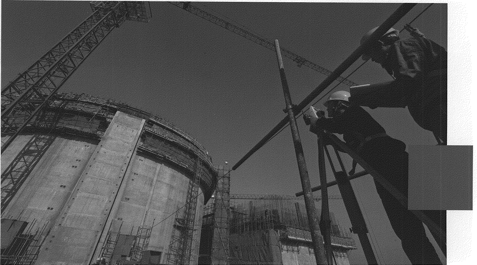
Fuqing nuclear power station under construction in China.
