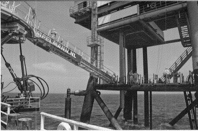
SMIT cooperated with the Delft University of Technology (TU Delft) in the development of the "Ampelmann" system that enables safe transfer of crews from ship to ship on open sea.
