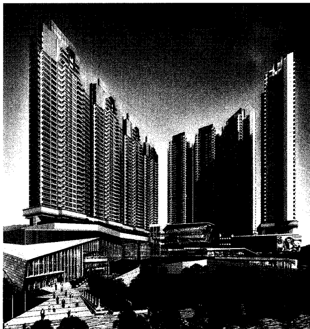
YOHO Midtown in Yuen Long consists of eight towers planned for completion by mid 2010.
