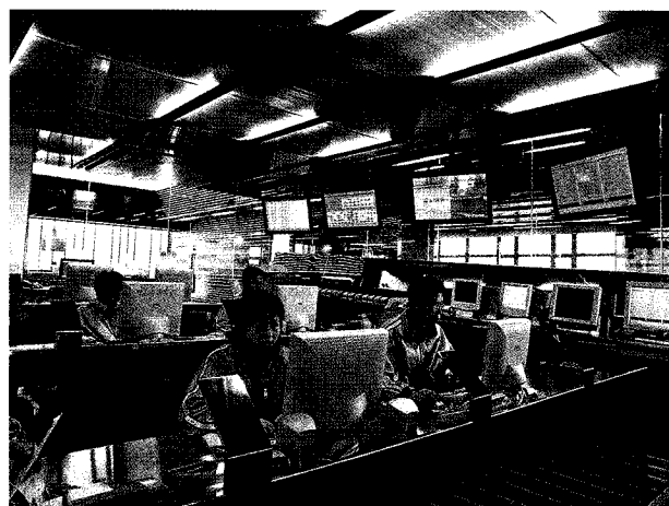
SUNeVision's iAdvantage provides world-class data centre facilities and service.
