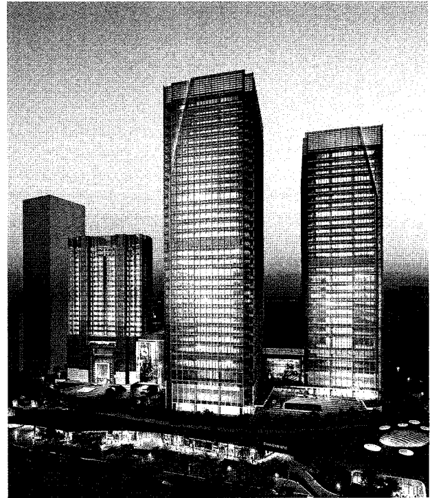
Shanghai ICC on Huai Hai Zhong Road will be a top-quality integrated development with convenient transport connections.
