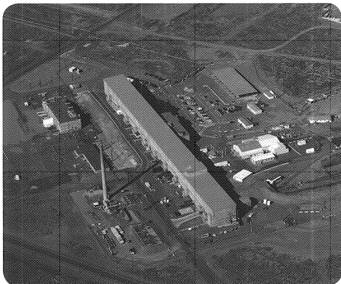
T plant at the Hanford site
