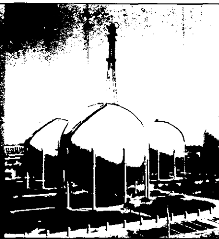
Natural gas sphere tanks
