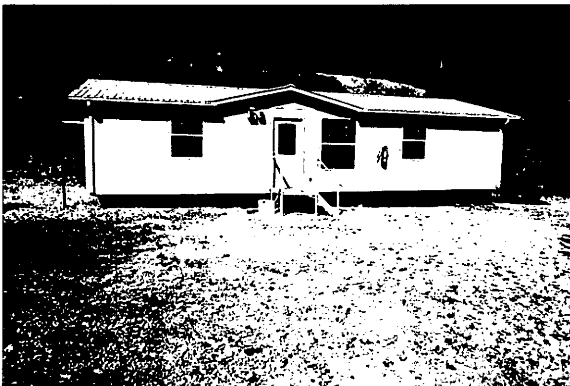
Figure 5: New all equipped offices
