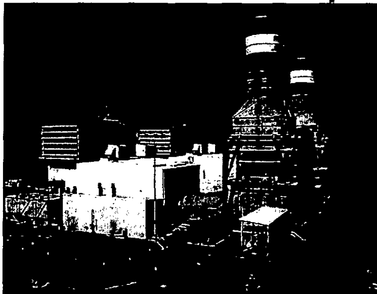
Oakey - 300MW Gas Fired Power Station
