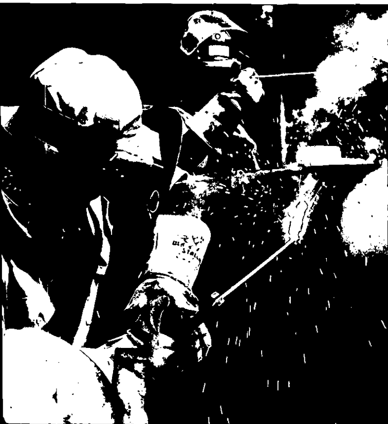
Welders work on 24-inch diameter pipe as part of the Battle Creek project. Working in a sensitive streamside area, crews moved and replaced two essential sections of pipe serving the Mist underground gas storage facility.
