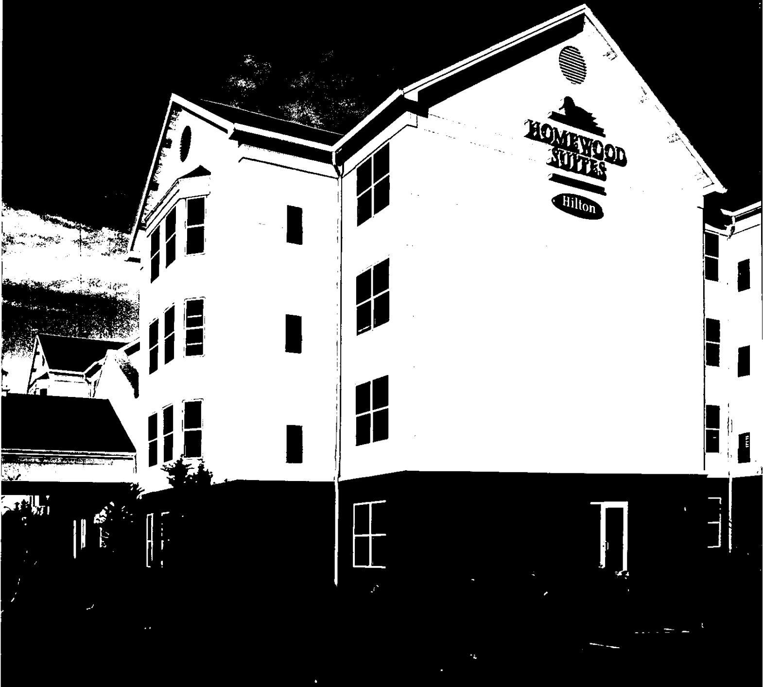
HOMEWOOD SUITES, PORTLAND, OR OPPOSITE: RESIDENCE INN, BOSTON TEWKSBURY, MA
