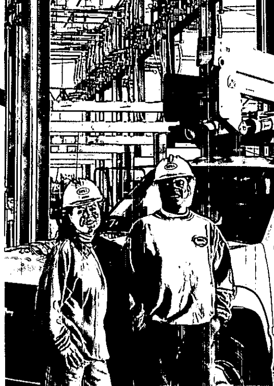
Allison Coate (left) and Quintin Gaddis play a valuable role in substation construction. DP&L built three new substations during 2006 to strengthen reliability and supply power to the region's growing areas.
