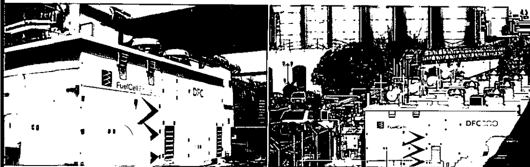
TST, Inc., Fontana, California Two DFC300A power plants provide 500 kilowatts to the aluminum smelter operations.
