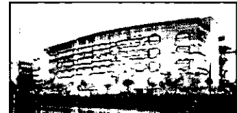
Quill Building 4 – DHL 2
