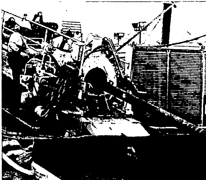
Drilling of the main gas pipeline at the horizontal directional drilling (HDD) site.
