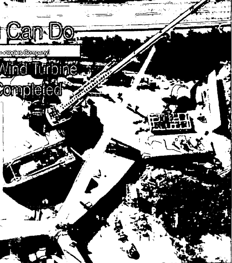
View of the 80 meter diameter rotors being assembled from the top of the 60 meter high tower
