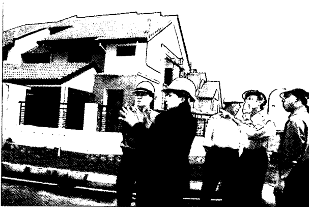
Quality inspections are conducted regularly at site
