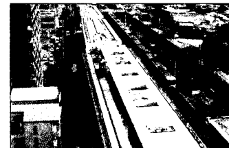
Elevation of railway track (Kachigawa)
