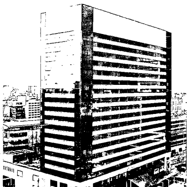
JR Shinagawa East Building
