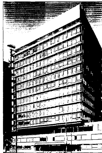
The existing 122 Leadenhall Street
