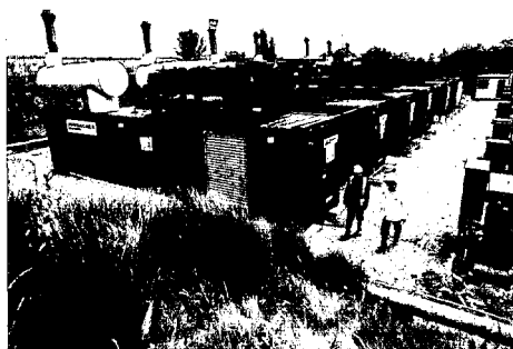
Above Renewable energy generation, Risley landfill site.
