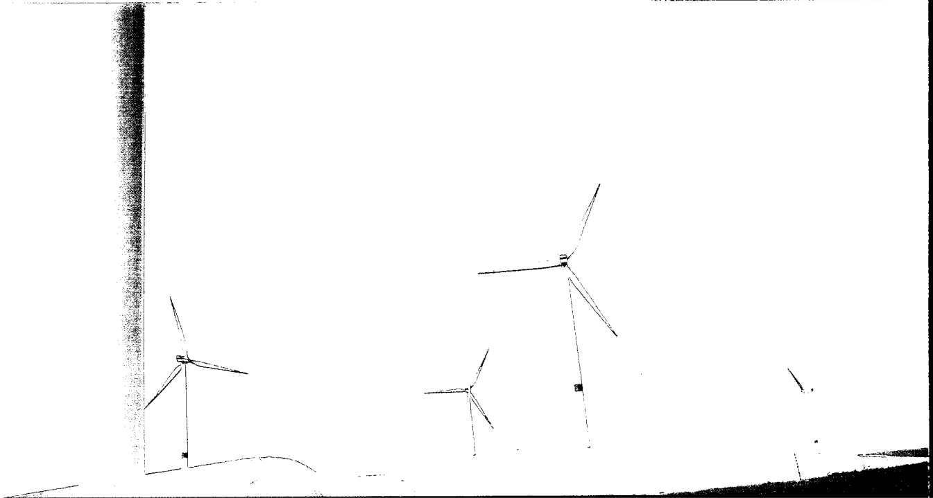
Installation of V80-2.0 MW wind turbines in Grossenerich, Germany
