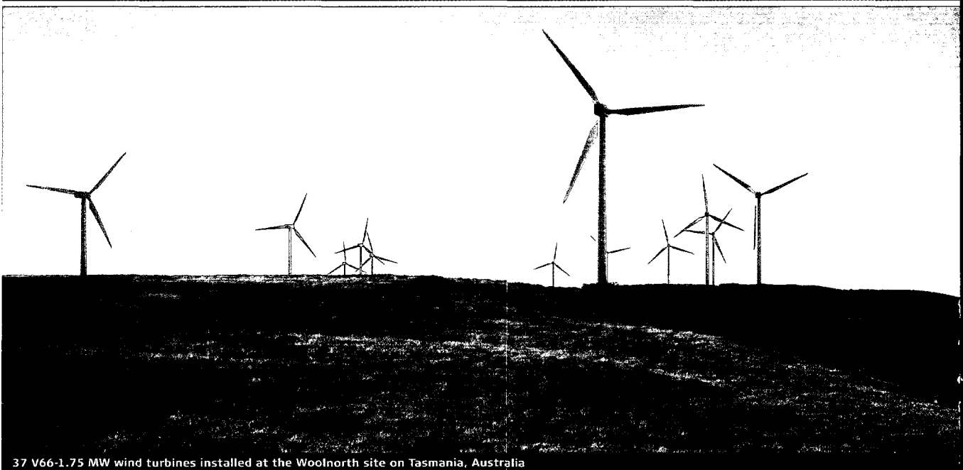
37 V66-1.75 MW wind turbines installed at the Woolnorth site on Tasmania, Australia
