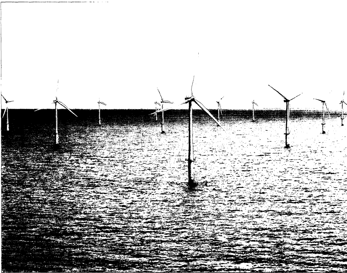
The offshore North Hoyle wind farm consisting of 30 V80-2.0 MW turbines has been set up approximately 7 km off the north coast of Wales.
