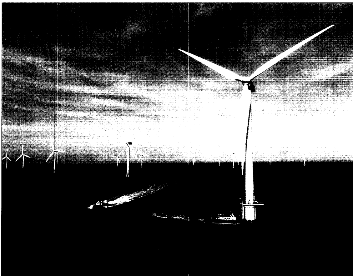
On the British market, Vestas has captured a large share of the offshore area. This market share is attributable in part to the delivery of a total of 60 V80-2.0 MW offshore wind turbines to the Scroby Sands and North Hoyle projects. The picture here shows wind turbines at Scroby Sands, approximately 3 km off the coast of Great Yarmouth in Norfolk, in the east of England.
