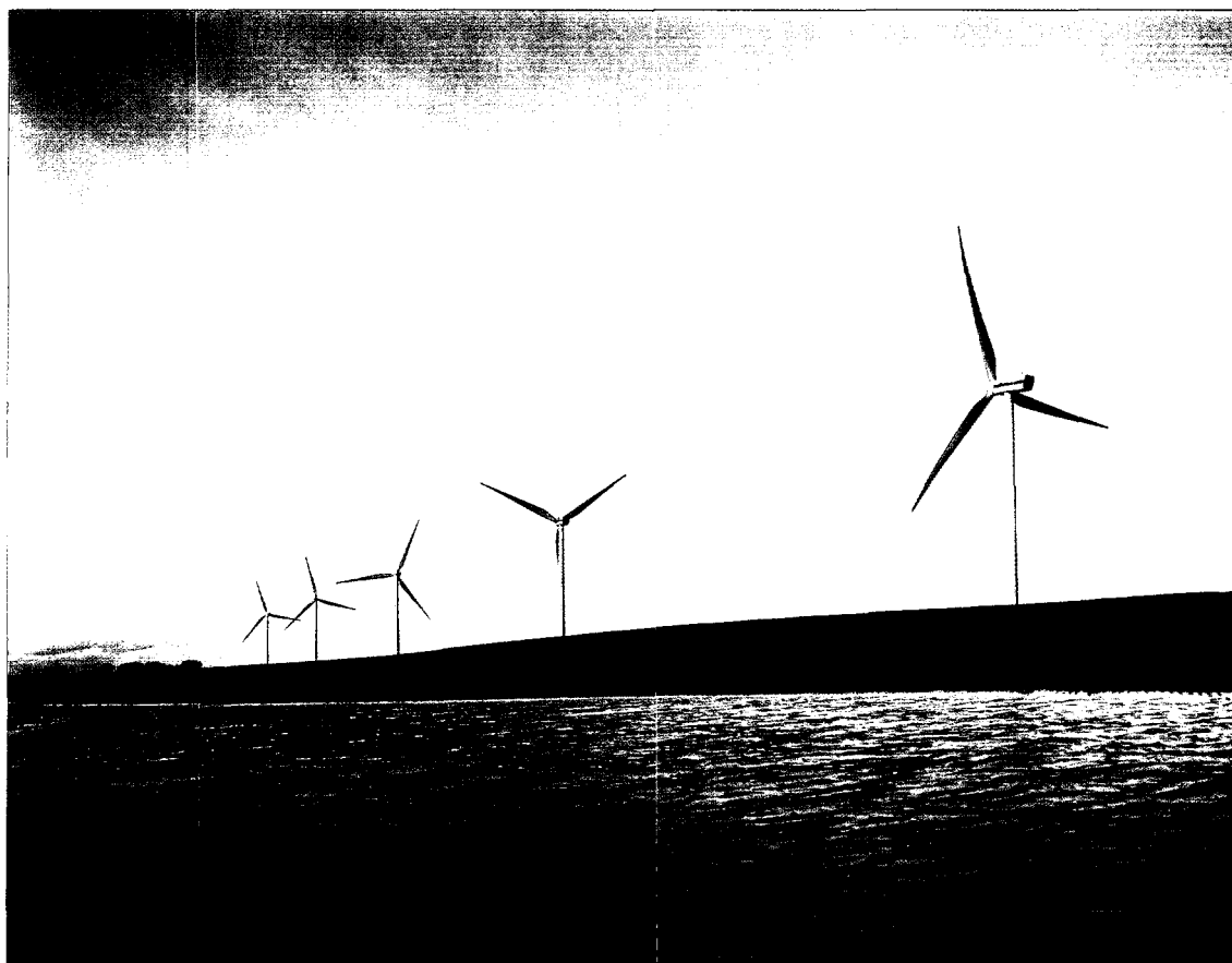
V80-2.0 MW wind turbines installed near Lemvig, Denmark.
