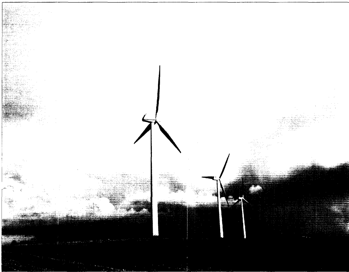
NM48-750 kW wind turbines installed in Funen, Denmark.
