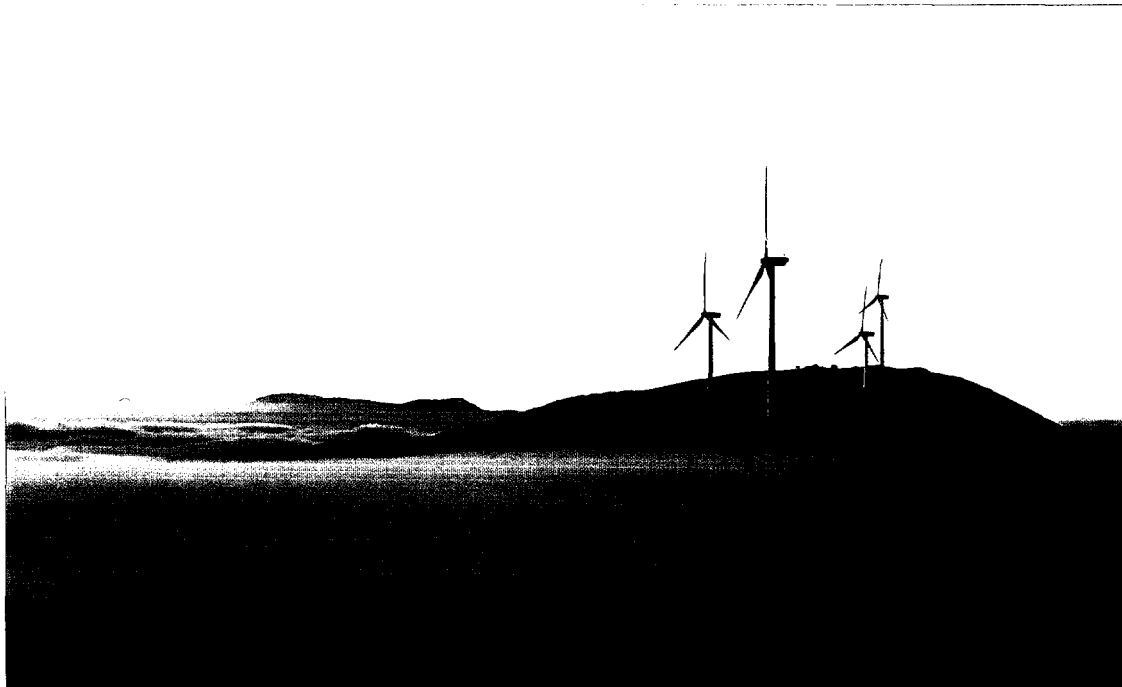
The Meroicinha site in Portugal consists of three V80-2.0 MW turbines and one V90-3.0 MW turbine.
