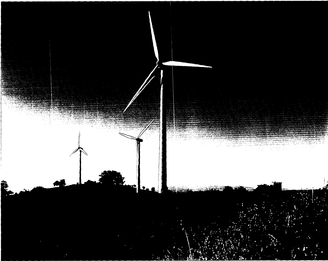
Eight V47-660 kW turbines erected at the Montemurro site in Italy.
