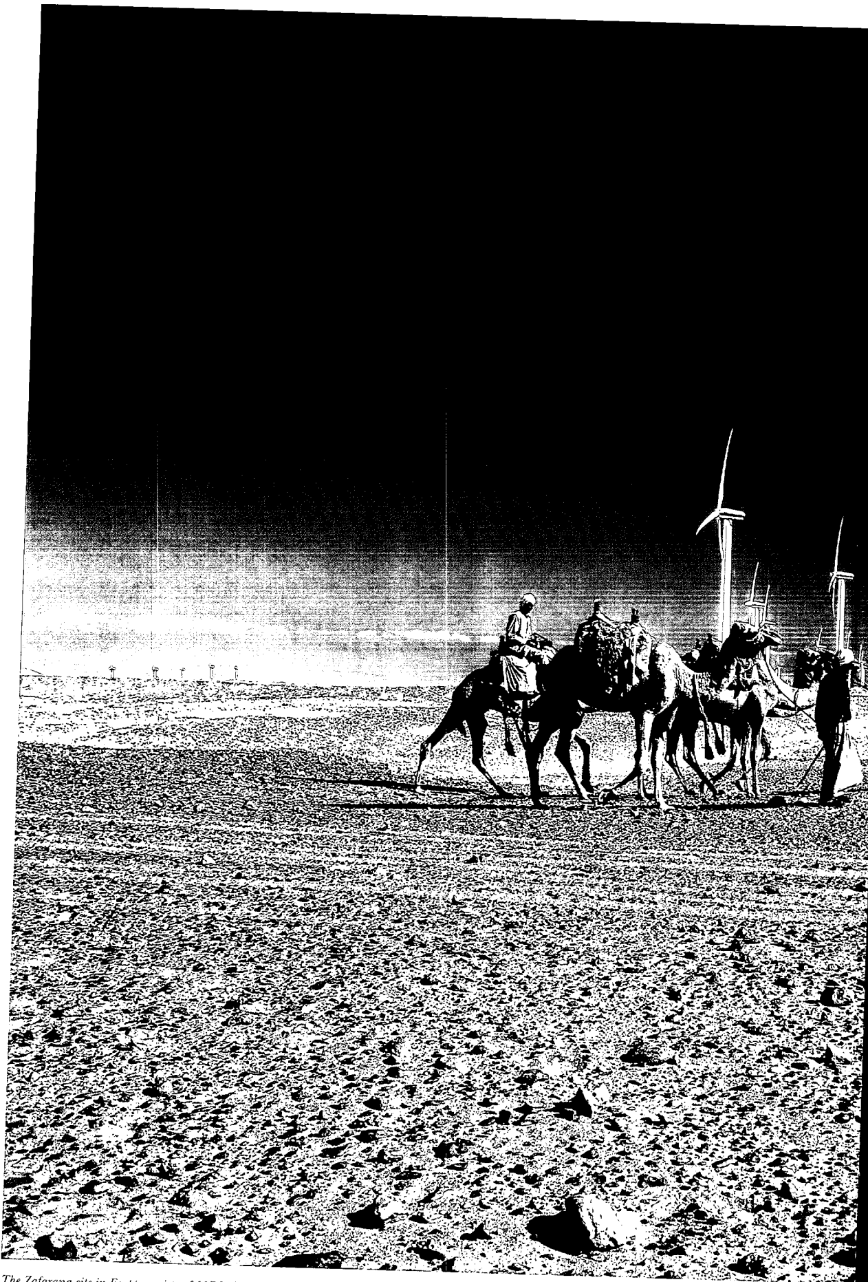
The Zafarana site in Egypt consists of 117 V47-660 kW turbines.
