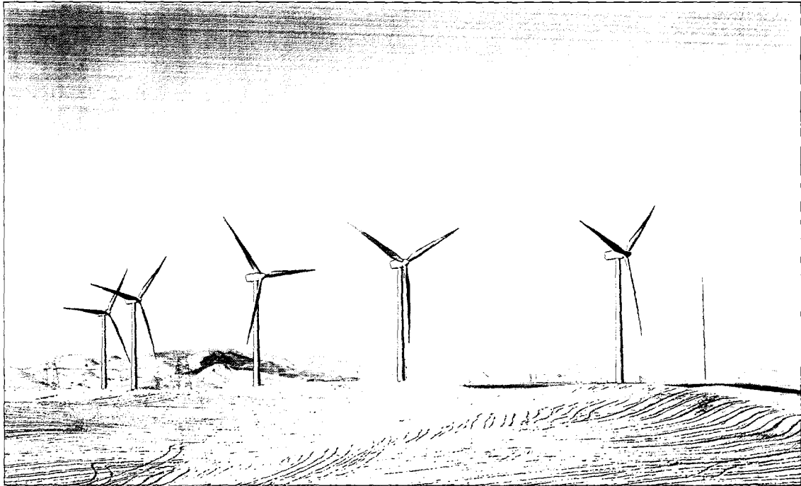
The High Winds project in the United States comprises eighty-one V80-1.8 MW turbines.
