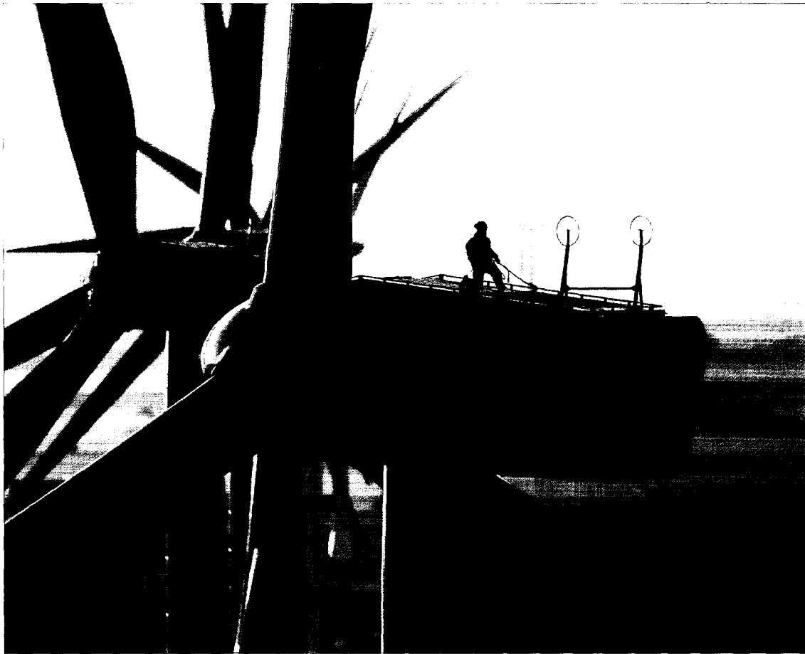
Thirteen V80-2.0 MW turbines installed at Reussenköge constituted the largest repowering project in Germany in 2003.
